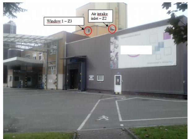
Fig. 8. Main noise sources Z2 and Z3.
